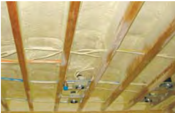
Figure 6. Fiberglass and cellulose insulation are usually installed in contact with the back of the drywall; the concern is that leaving a space there allows convective air currents to degrade the insulation's thermal performance. Because closed-cell foam is unaffected by air movement, the space between it and the drywall is not a problem.
